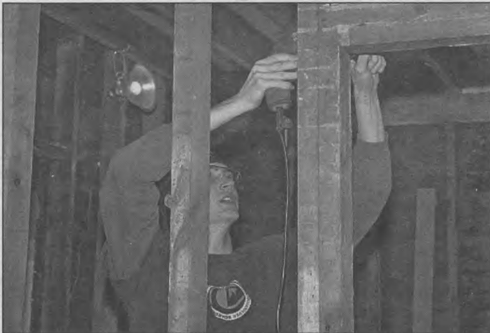
Sophomore Tyler Hoyle builds a door frame in a house damaged by flooding in Cedar Rapids, Iowa during the week of fall break. Photo submitted.
